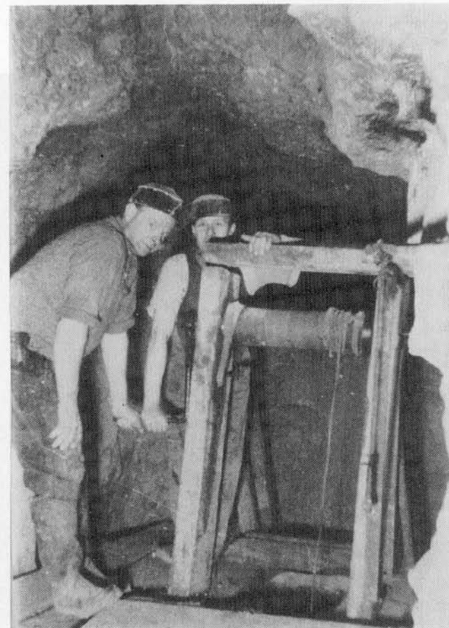
6. 93 ftm level: stowes at the top of a clean-up winze to the bottom of a wing deposit.
