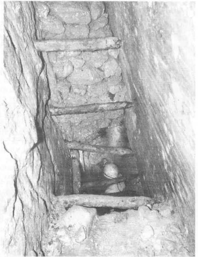
Winze leading to levels below 97m.
