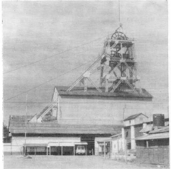
Gifford Shaft headstocks on Champion Reef Mine. 6563 feet deep, it leads via sub-levels to a total depth of 10,300 feet below collar.
