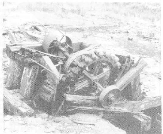
Plate 5 (below). Nantiago: Remains of the Pelton wheel with settling tanks in the background.
