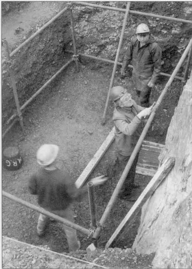
Plate.1 Copa Hill 1989-91. Installing shoring.
