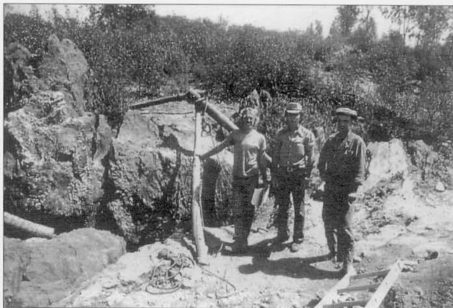
Plate 5. Chinflon - Mine 4B during excavation.
