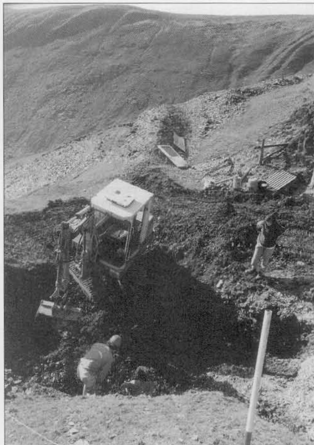
Plate 3. 1993. Site during machining, view to west.
