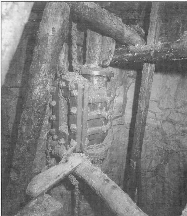
(Below) Top valve box of the lift pump.
