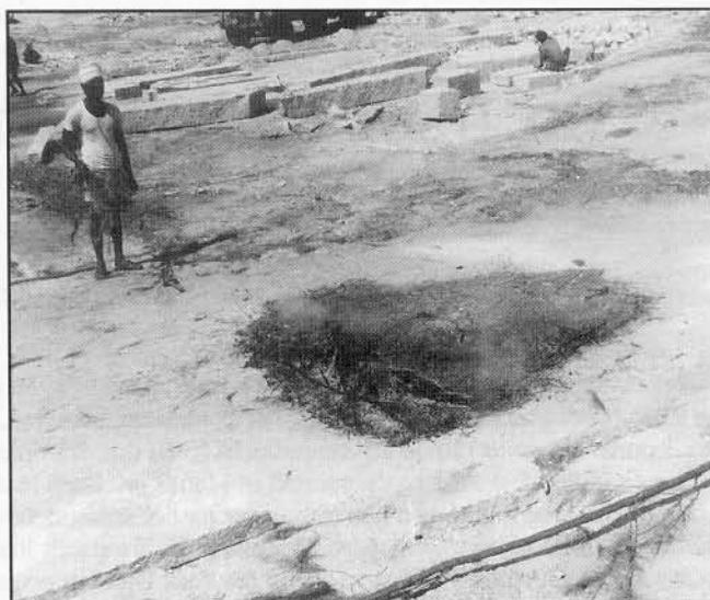
Plate 6. (above). Fire of brushwood burning over the crack and controlling its spread. Note the granite pillars in the background split from a thick slab.
