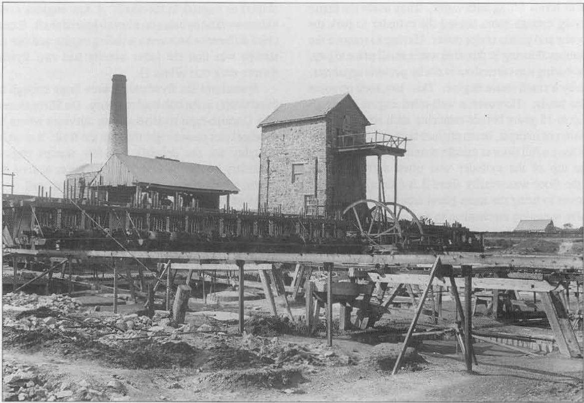
Plate 1. A typical stamps engine at Wheal Grenville, near Camborne(c1904) showing the twin flywheels, separated chimney stack and the long row of tin stamps each side. Tie rods and glands have been added to strengthen the bob wall.
