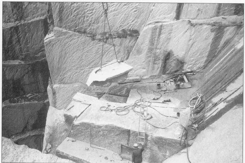
Plate 6. Lifting a block with 'dog' hooks. Note face behind, showing characteristic marks of jet-channelling, March 1993.
