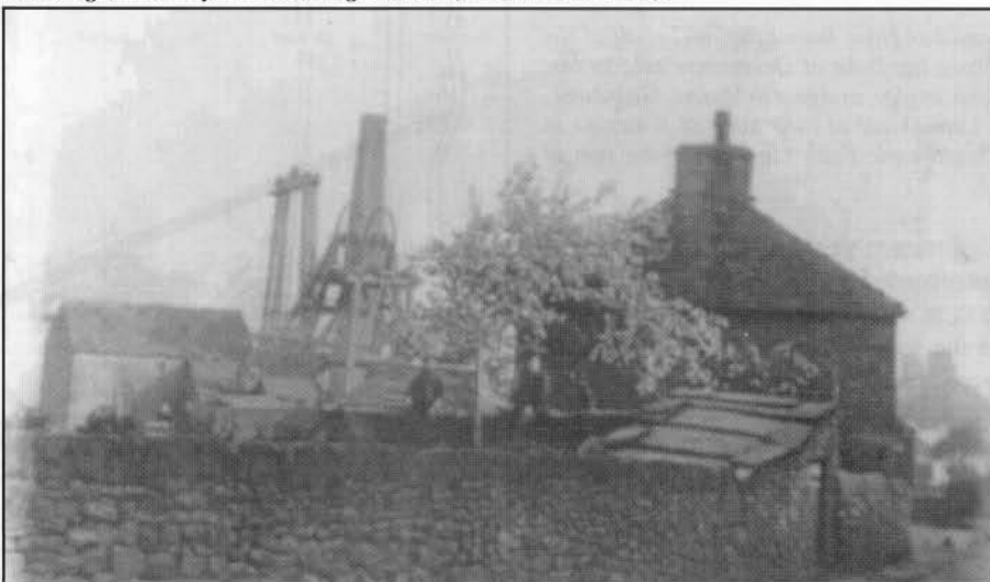
Plate 2. Waterloo (Gisbourne's) Colliery Pithead from Old Road, showing headframe, shearlegs, chimney and winding-house. (Private Collection).
