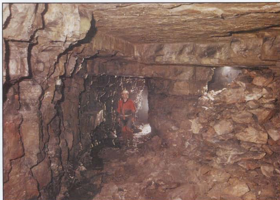
Plate 3. Deep Ecton Sough, with the 1774 re-driving to the left and the blocked original course to the right.
