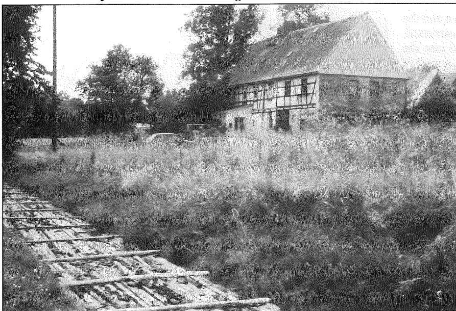
Plate 1. A modern view of the covered ditch that supplies water from the Grosshartmannsdorf reservoirs to the Freiberg district.
