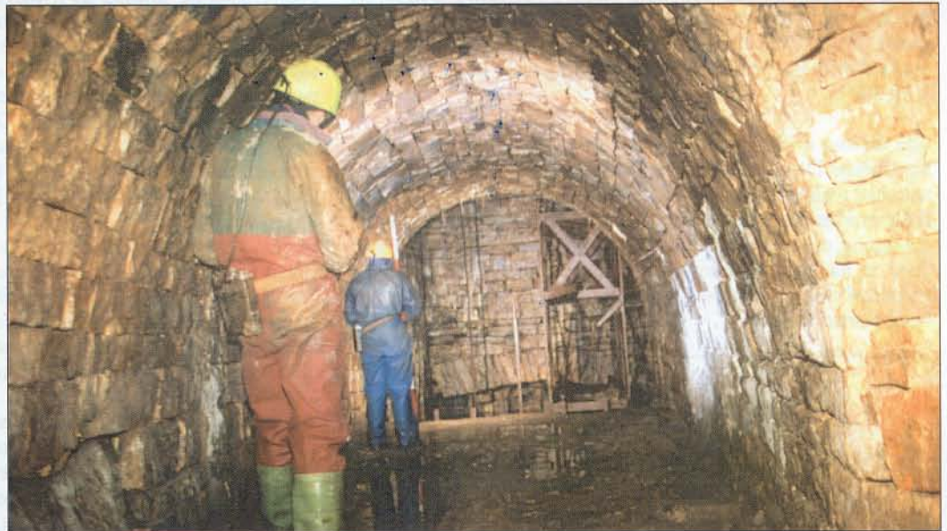
Plate 1 (top left). Pump Spear - Old Gang Engine Chamber.
