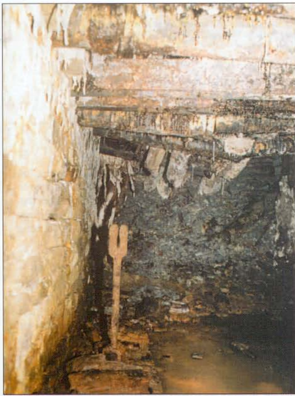
Plate 1 (top left). Pump Spear - Old Gang Engine Chamber.
