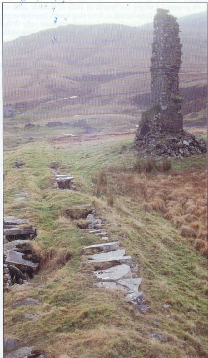
Plate 7 (below). Woodhead south smelter chimney and flue.
