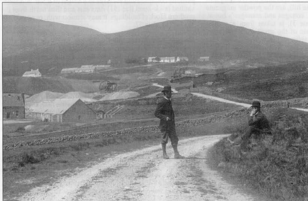
Plate 3. Woodhead Lead Mine c.1890s showing the waterwheel and extensive waste tips. Taken from the east. (Source Carsphairn Heritage Centre).
