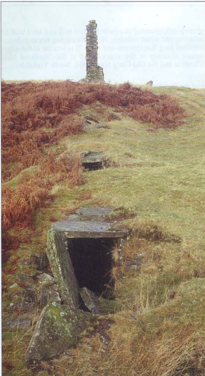
Plate 6 (below). Woodhead Mine smelter flue with chimney.
