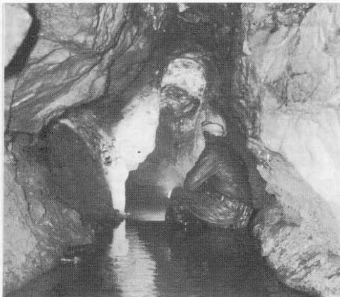
2. Typical section with picked top section in shale, limestone bed across the middle and shale below in the footings.
