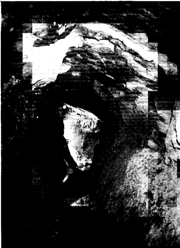
3. Section with limestone bed in the roof and shale walls. Scattered shot holes in the roof; picked shale walls.
