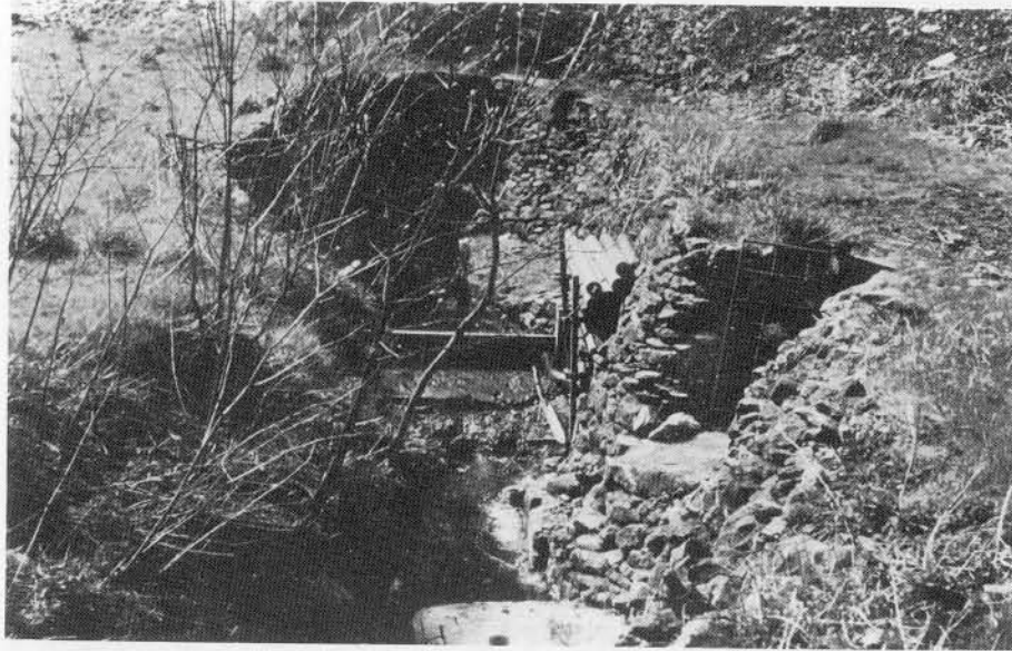
1. Slop Moll (centre) and Peakshole Sough entrance (right).
