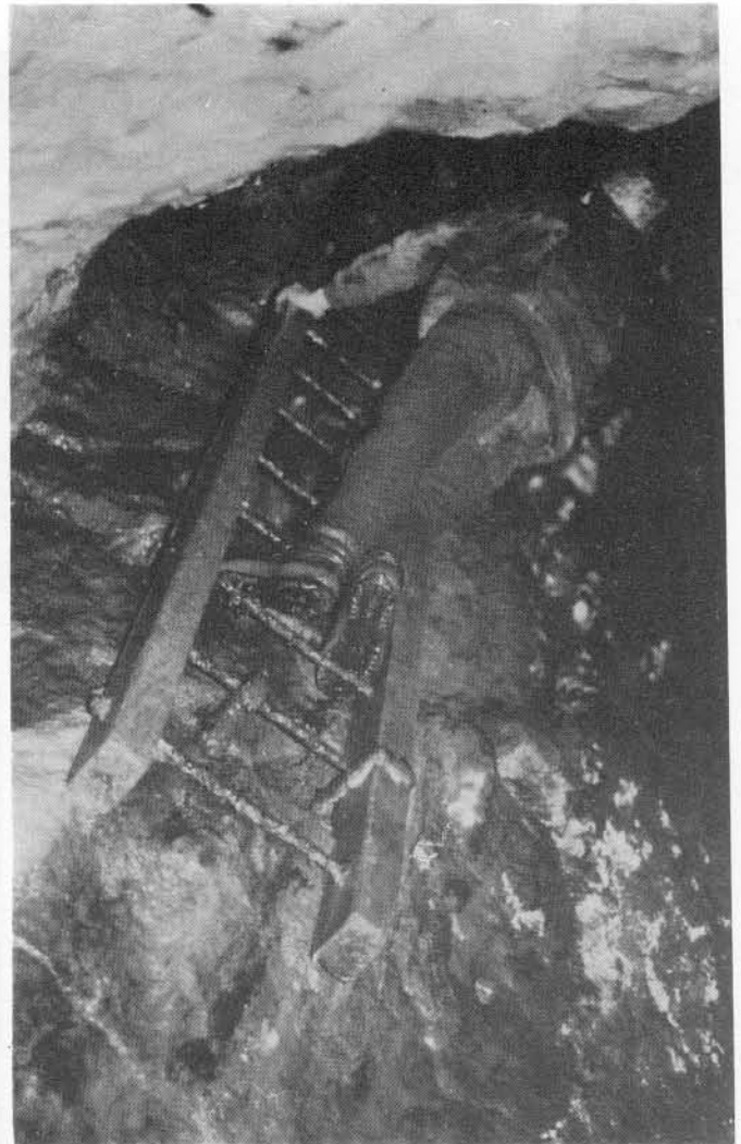
6. Ladderway through stopes above No. 1 Level.
