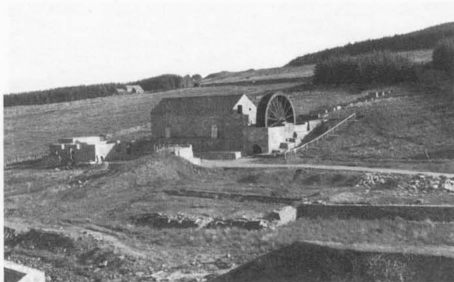
Plate 1. Overall view from the northeast before excavation: bridge abutment in foreground, washing floor and Brunton Buddles in the middle distance, with mechanised dressing mill behind.
