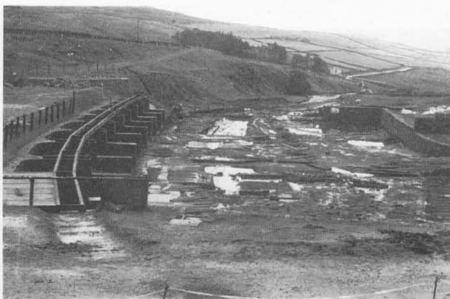
Plate 2. Overall view of washing floor from the east during 1985 excavations.
